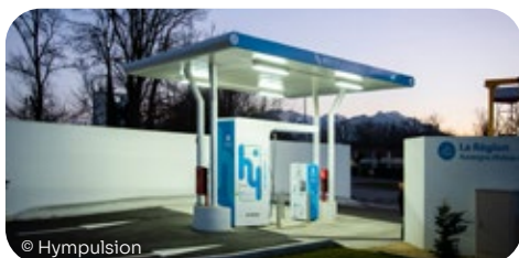
Station Himpulsion de Chambéry
